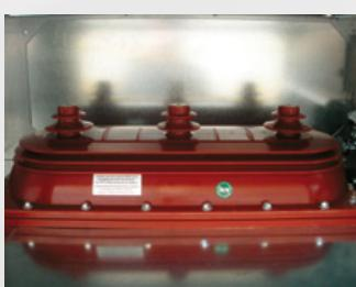
The *on-load* switches IM6 type, with resin envelop, are filled with hexa-fluoride (SF<sub>6</sub>) as dielectric insulation and interruption. Its position creates a separation between the bus bars compartment and the main equipment compartment.
