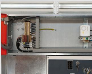
This compartment is used to set the auxiliary command and control equipments, such as protection relay, control buttons, signaling lamps, terminal boards, etc..
