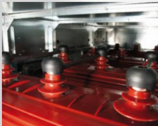
In the bus bars compartment are placed the three main bus bars of the system. This sector is completely isolated from the main equipment compartment, allowing a total safety access to this one, with main bus bars in tension too, according to the classification LSC2A.
