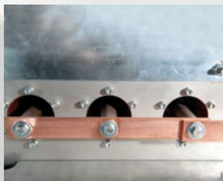
In order to check the insulation of the cable or to search failures you can enter a voltage across the dedicated loops by closing the earth switch and opening the mobile connection of grounding.
