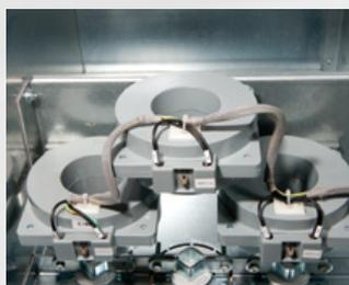
They provide to the relay the current signal to be elaborated and the necessary energy to power it and the shunt opening release. They can have a primary current of 50A, 100A or 150A.
